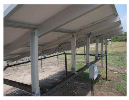
The solar panels from below. The panel control was bolted to the metal frame.
