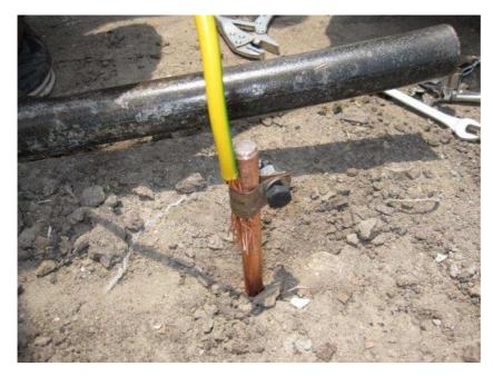
The earth rod with an improvised clamp, it was forced into the ground so that it is no longer visible.
