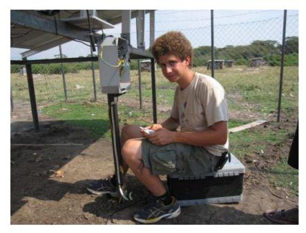
Valentin Koestler having been responsible for the installation of the solar system is doing electrical connections in the control box for the solar panels.
